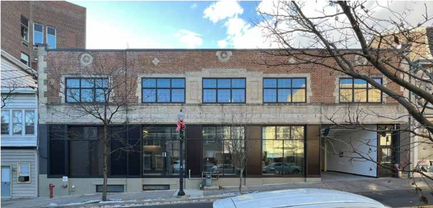
Image 44: Enlarged View, 320-324 West Fourth Street, Bethlehem, PA. Image taken by Spillman Farmer Architects on December 5, 2025.
