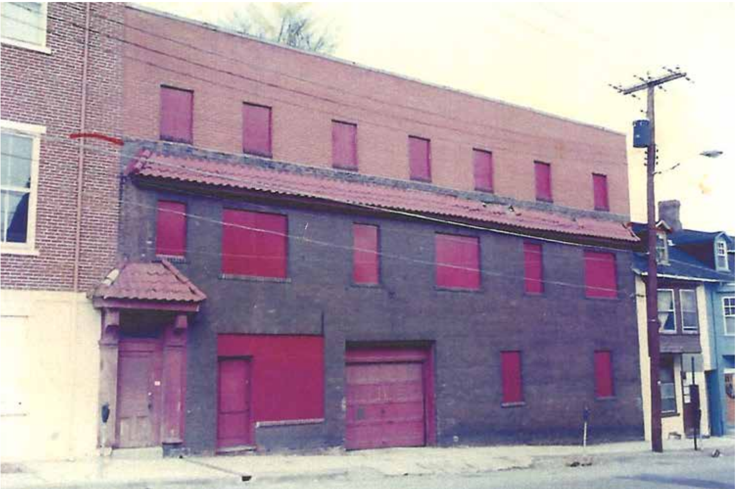
Image 29: 335-339 West Fourth Street, South Elevation; circa 1970-1985; Photograph provided by New Bethany
