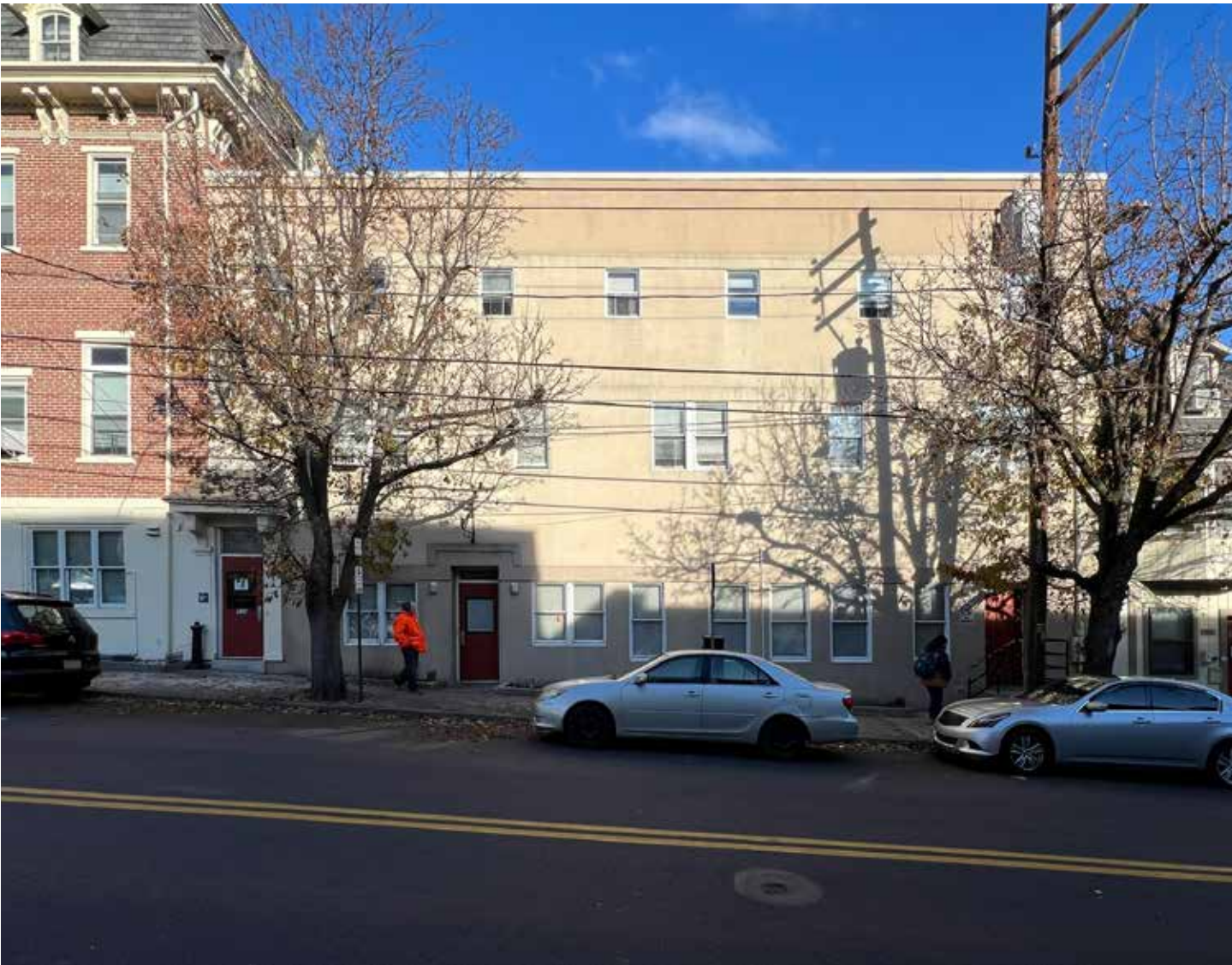
Image 37: Enlarged View, 339-335 West Fourth Street, Bethlehem, PA. Image taken by Spillman Farmer Architects on December 5, 2025.
