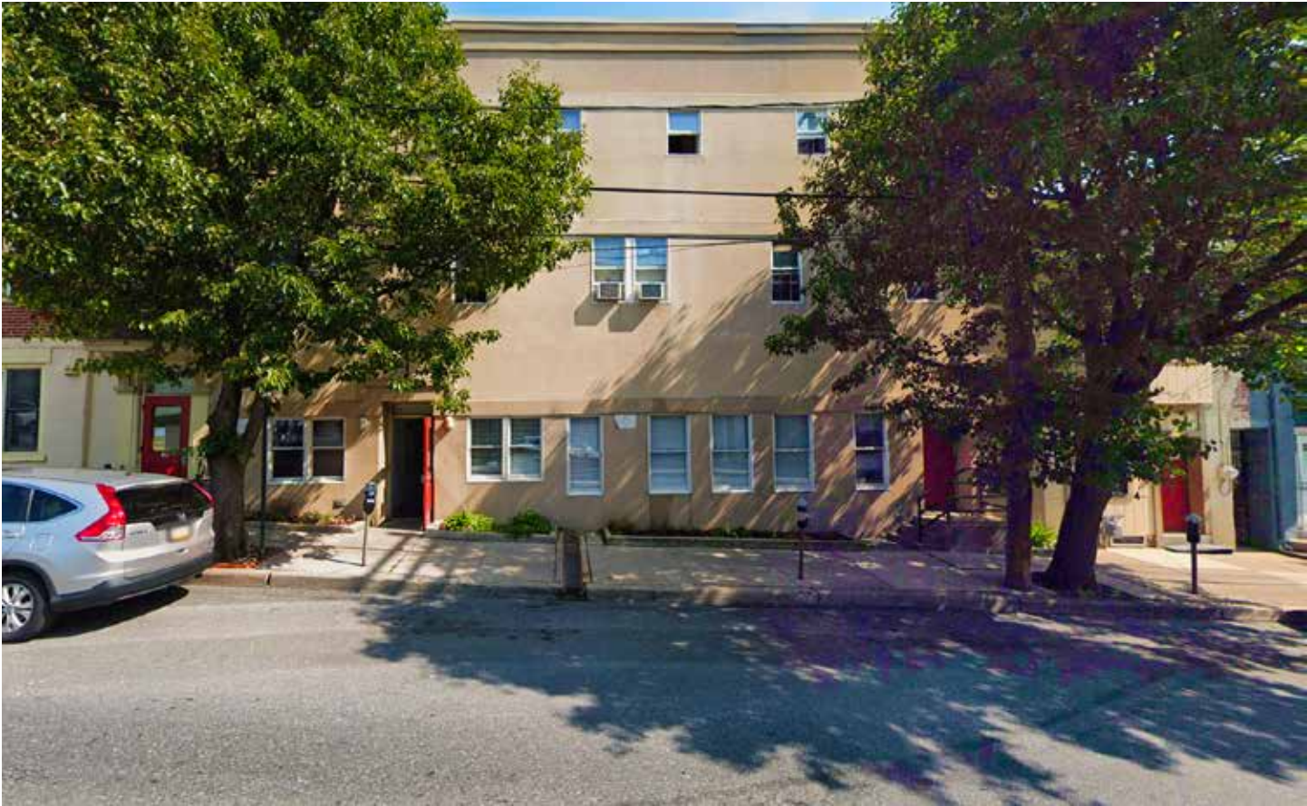
Image 2: 335-339 West Fourth Street, South Elevation; Image from Google Street View, July 2019.
