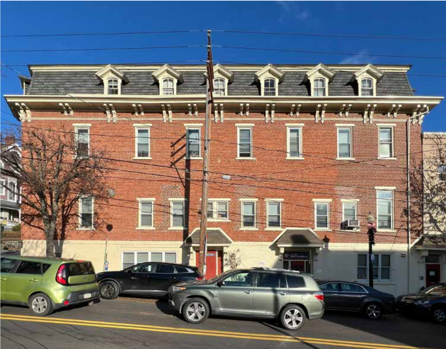
Image 39: Enlarged View, 341-345 West Fourth Street, Bethlehem, PA. Image taken by Spillman Farmer Architects on December 5, 2025.
