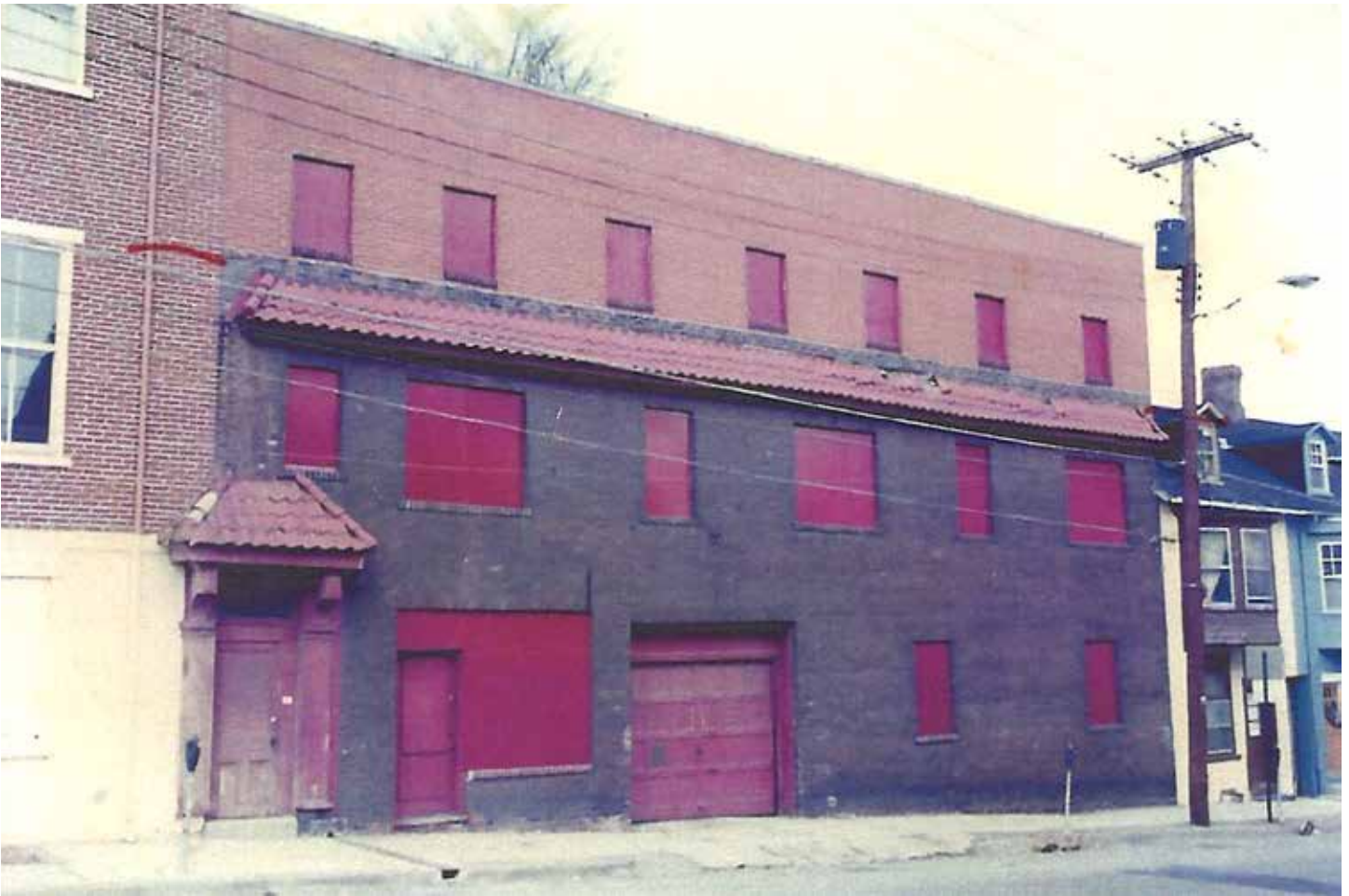
Image 32: 335-339 West Fourth Street, South Elevation; circa 1970-1985; Photograph provided by New Bethany
