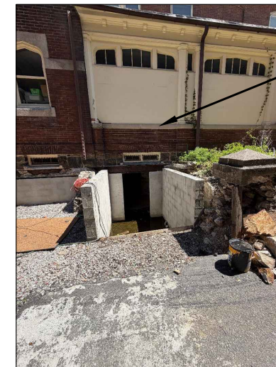
CURRENT CONDITION LOOKING TOWARD EXISTING BASEMENT OPENING
