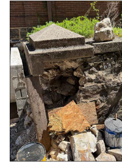
CURRENT CONDITION REAR WALL - LOCATION OF NEW STAIR
