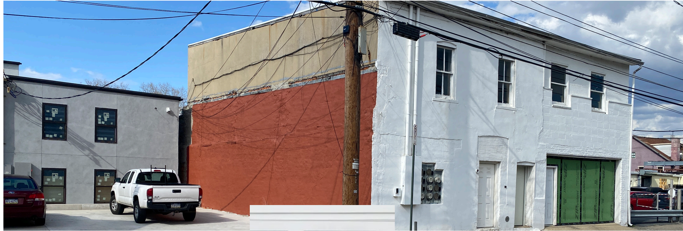
Partially painted, parged stucco West Facade at Property Line / Parking Lot
