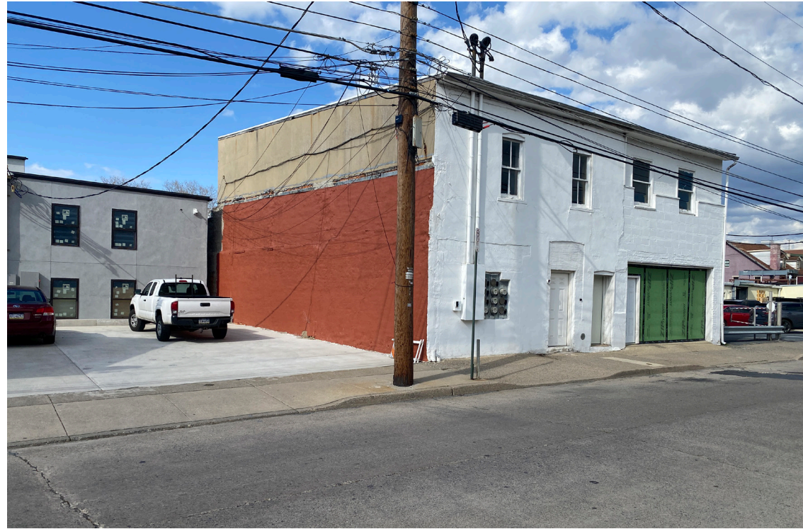
Partially painted, parged stucco West Facade at Property Line / Parking
