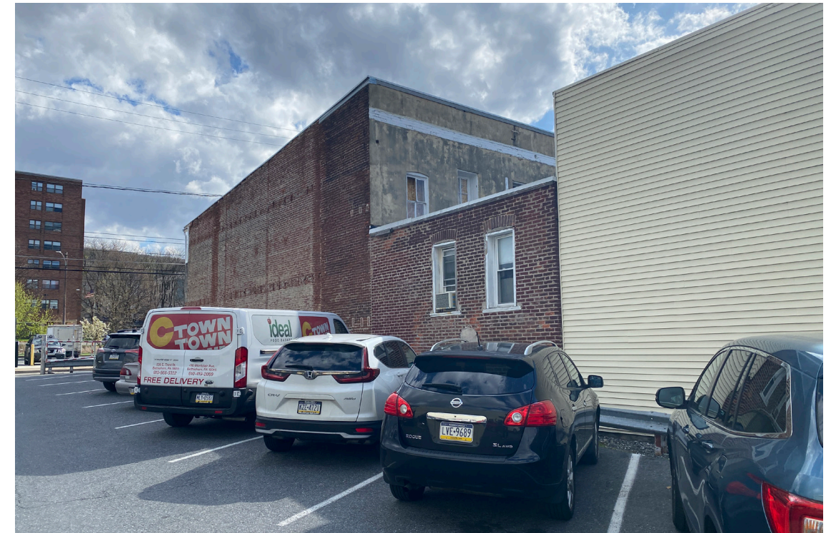
East Facade (exposed brick) and stucco at upper level - partial elevation
