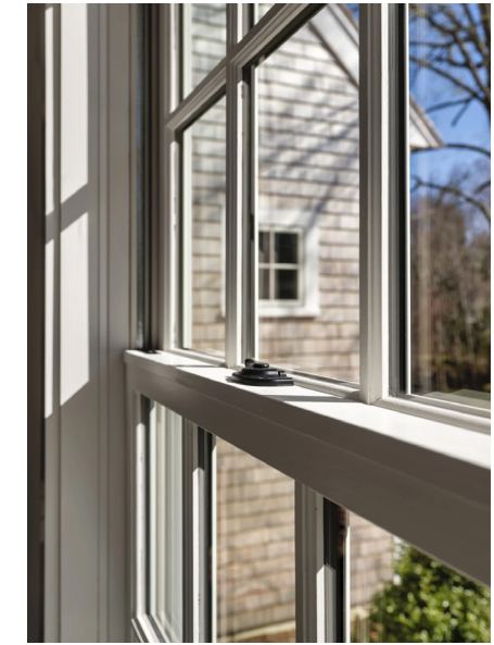
Proper meeting rail and simulated divided lite profiles at windows.
