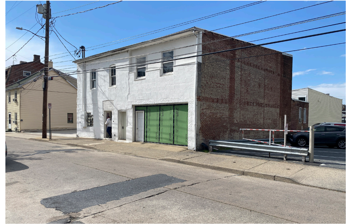
East Facade (exposed brick) on property line at Parking Lot
