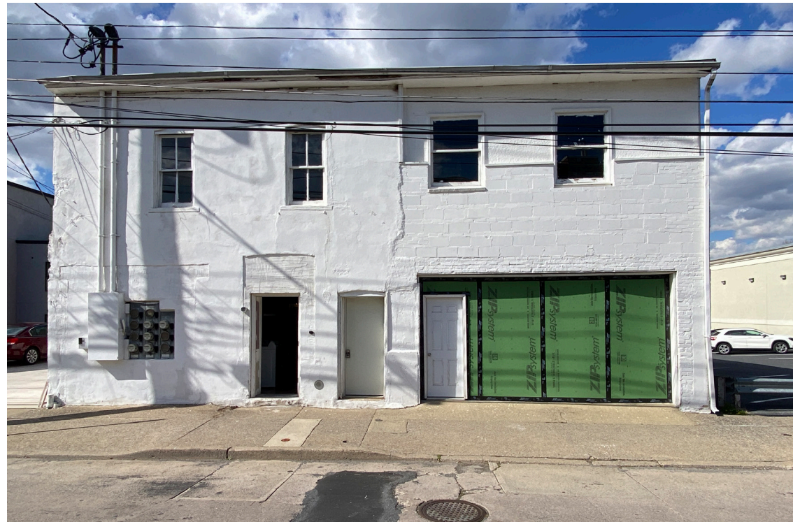
211 Mechanic Street - South Facade
